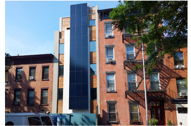
Solar PV Building Facades: Park Slope, NY
