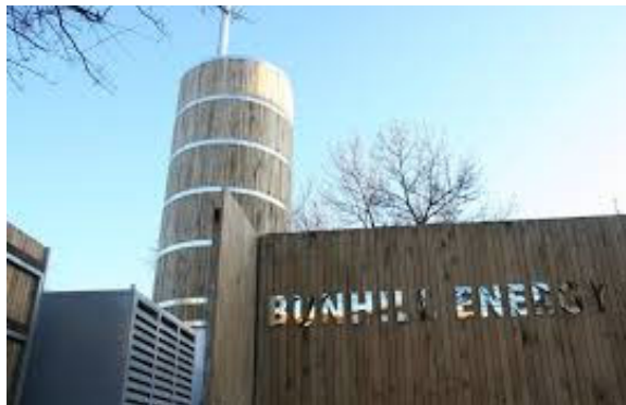
District Energy Systems & Neighborhood Shared Storage Bunhill Energy Centre | London
