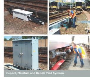
Inspect, Maintain and Repair Yard Systems
