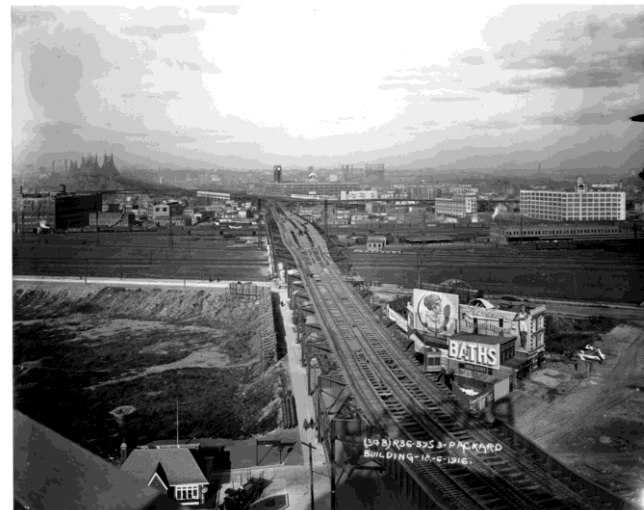
View of 7 line & Queensboro Bridge (1916)
