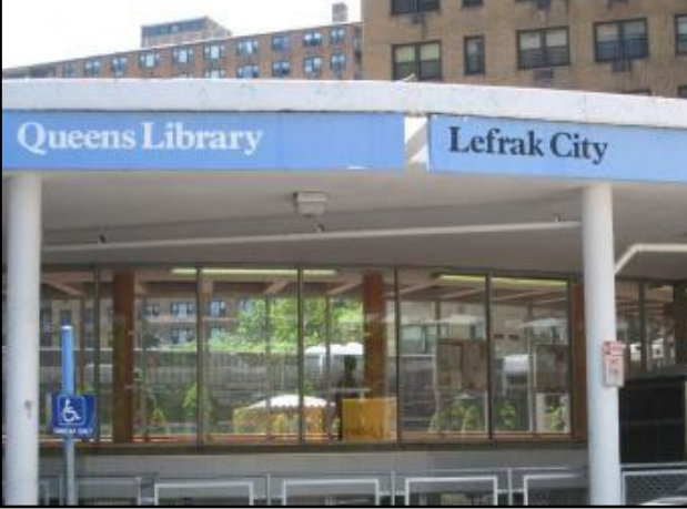
LeFrak City (1971) LeFrak City is a 40-acre complex of rental housing and offices with its own public library, post office, and sports facilities. A recent renovation installed solar panels on the roofs of 20 apartment towers.
