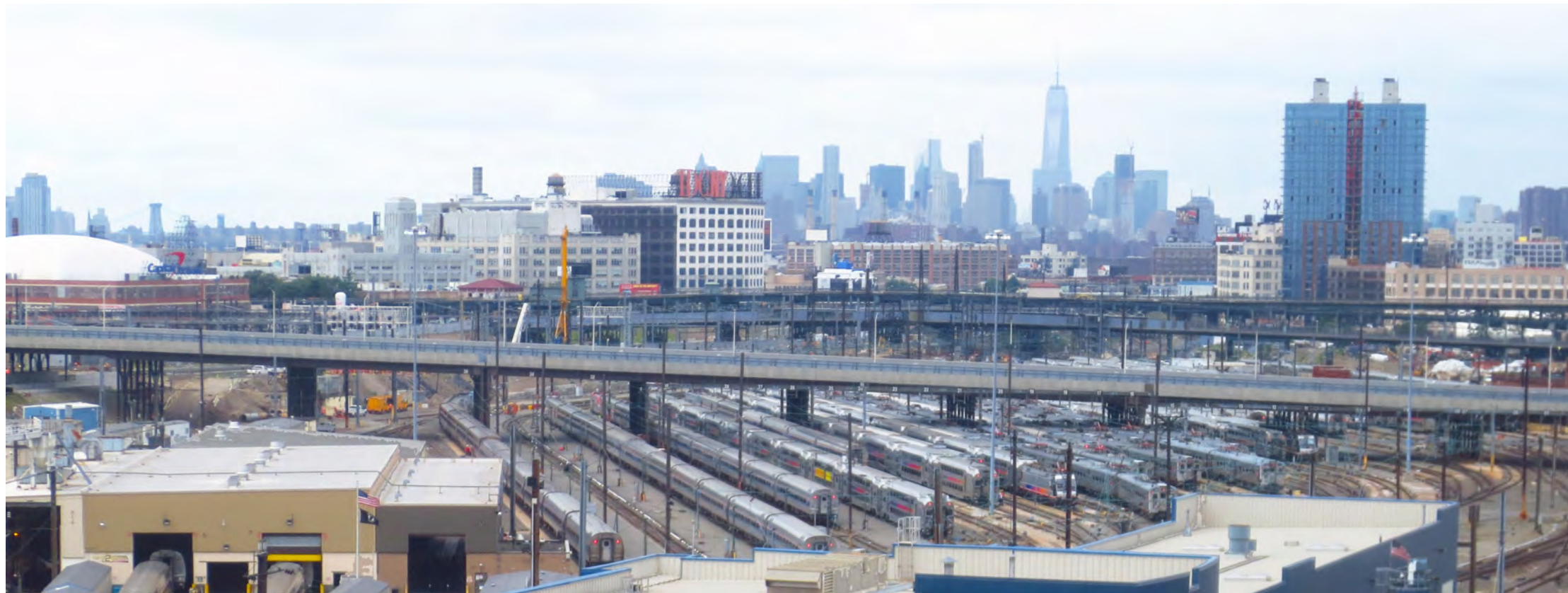
FIGURE 1.2: SUNNYSIDE YARD: EXISTING CONDITION
