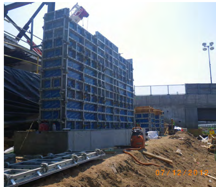
FIGURE 3.43: INTERNALLY TIED FORMWORK
