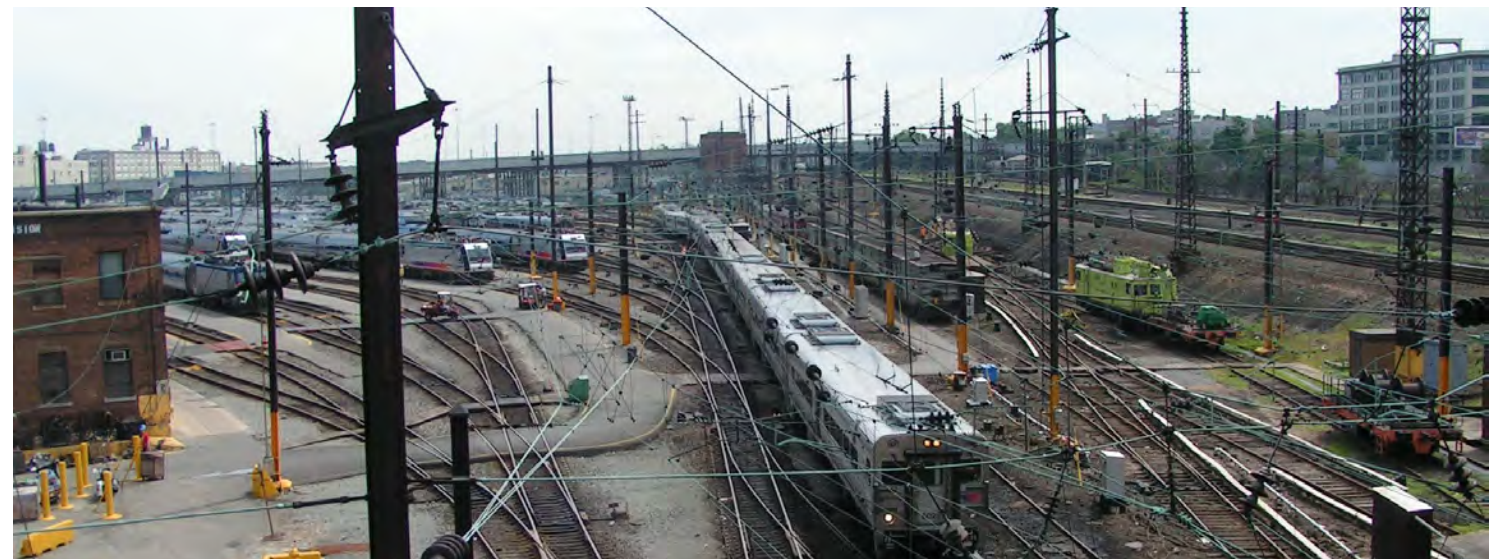
FIGURE 3.2: SUPPORT WIRES SPANNING SUNNYSIDE YARD
