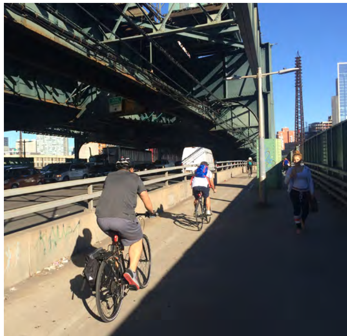
FIGURE 2.45 BIKE PATH / ED KOTCH QUEENSBOROUGH BRIDGE
