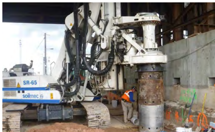
FIGURE 3.42: LOW HEADROOM PILING RIGS
