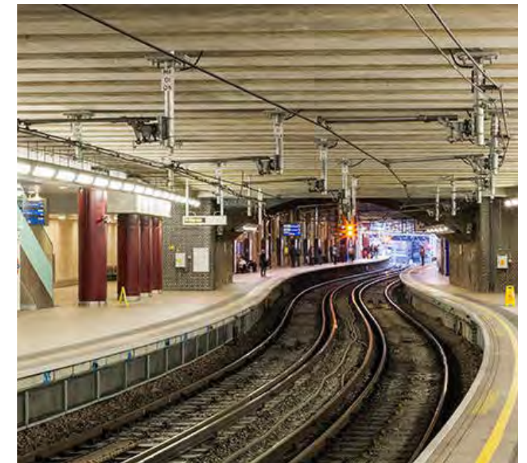
FIGURE 3.45: CATENARY MOUNTED UNDER DECK
