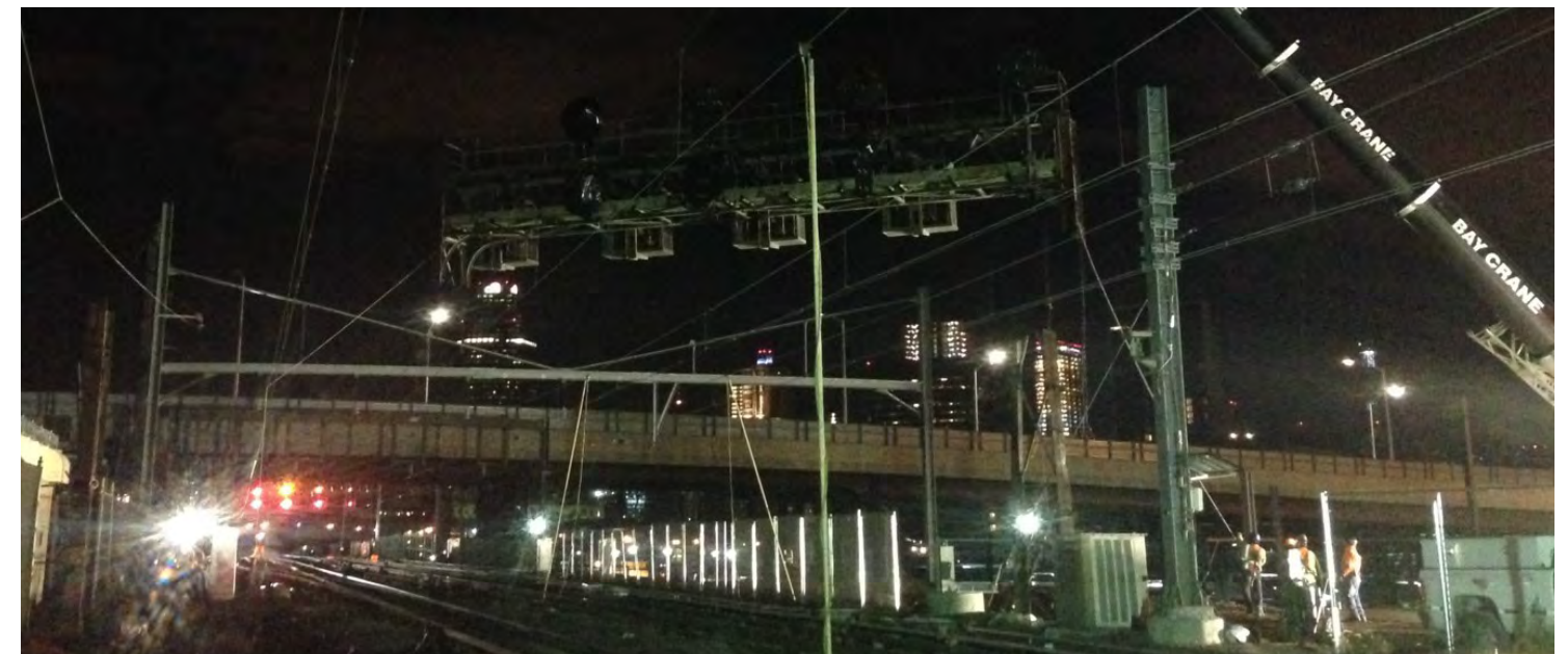
FIGURE 3.44 SIGNAL BRIDGE INSTALLATION
