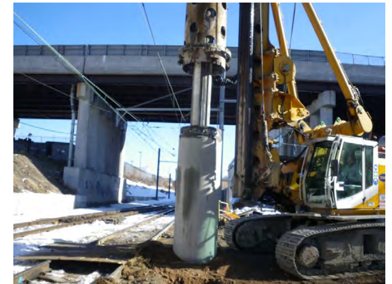
FIGURE 3.33 :SECANT PILES
