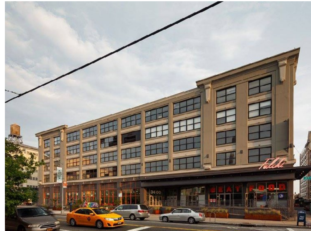
The Falchi Building Office example in LIC IBZ
