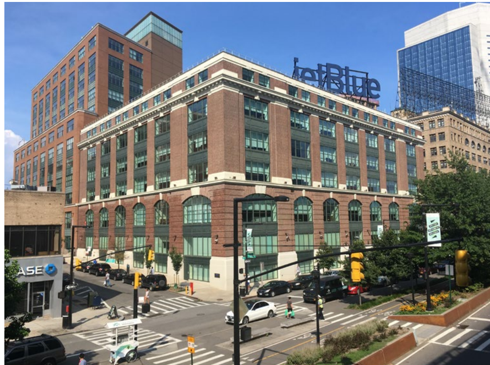
The JetBlue Building Office example in LIC
