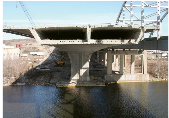
Figure 9 - Precast Concrete Segmental Girder
