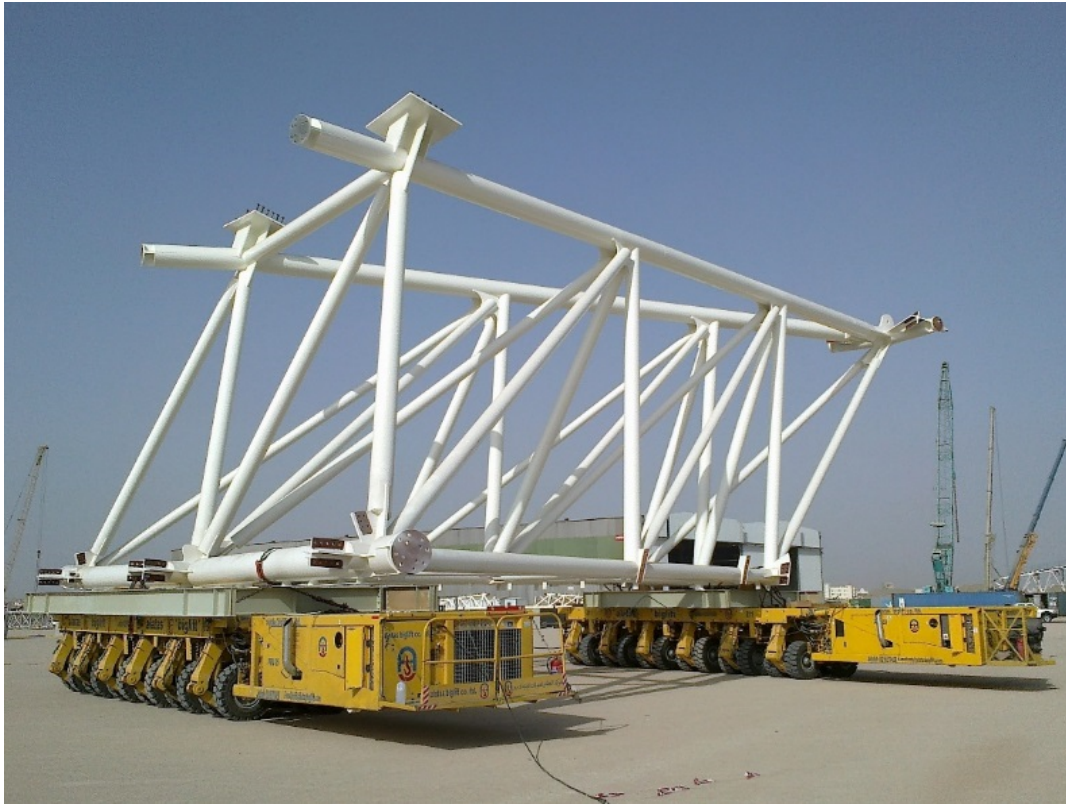
Figure 34: SPMTs at Work (Source: Alatas Big Lift)
