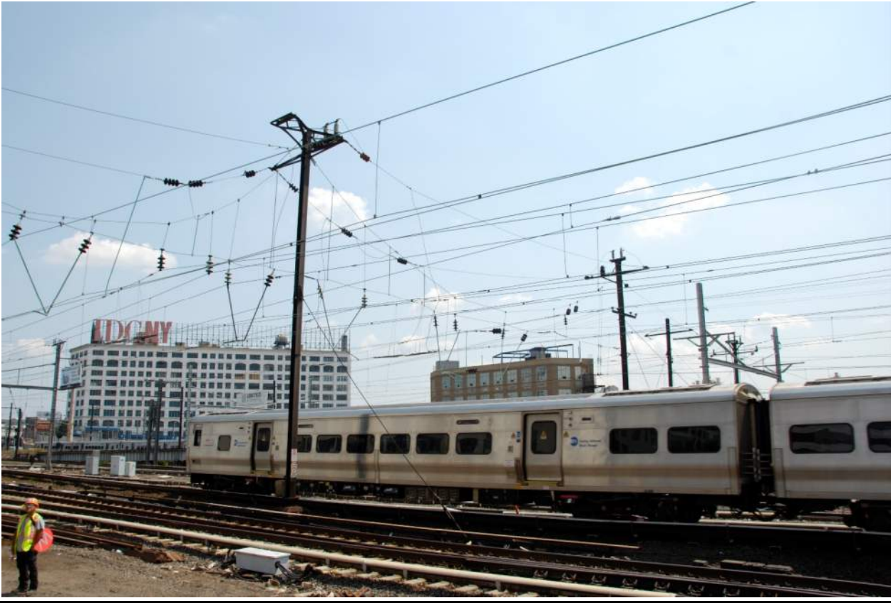
Zone 3 – X Catenary Structure (1):
