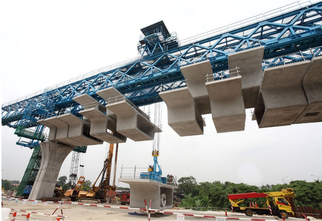
Figure 33: Launching Gantry (Source: Huada Crane)
