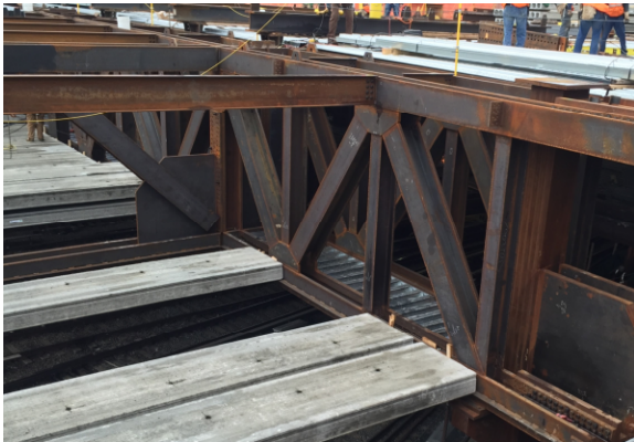
Figure 13 - Truss and Plank
