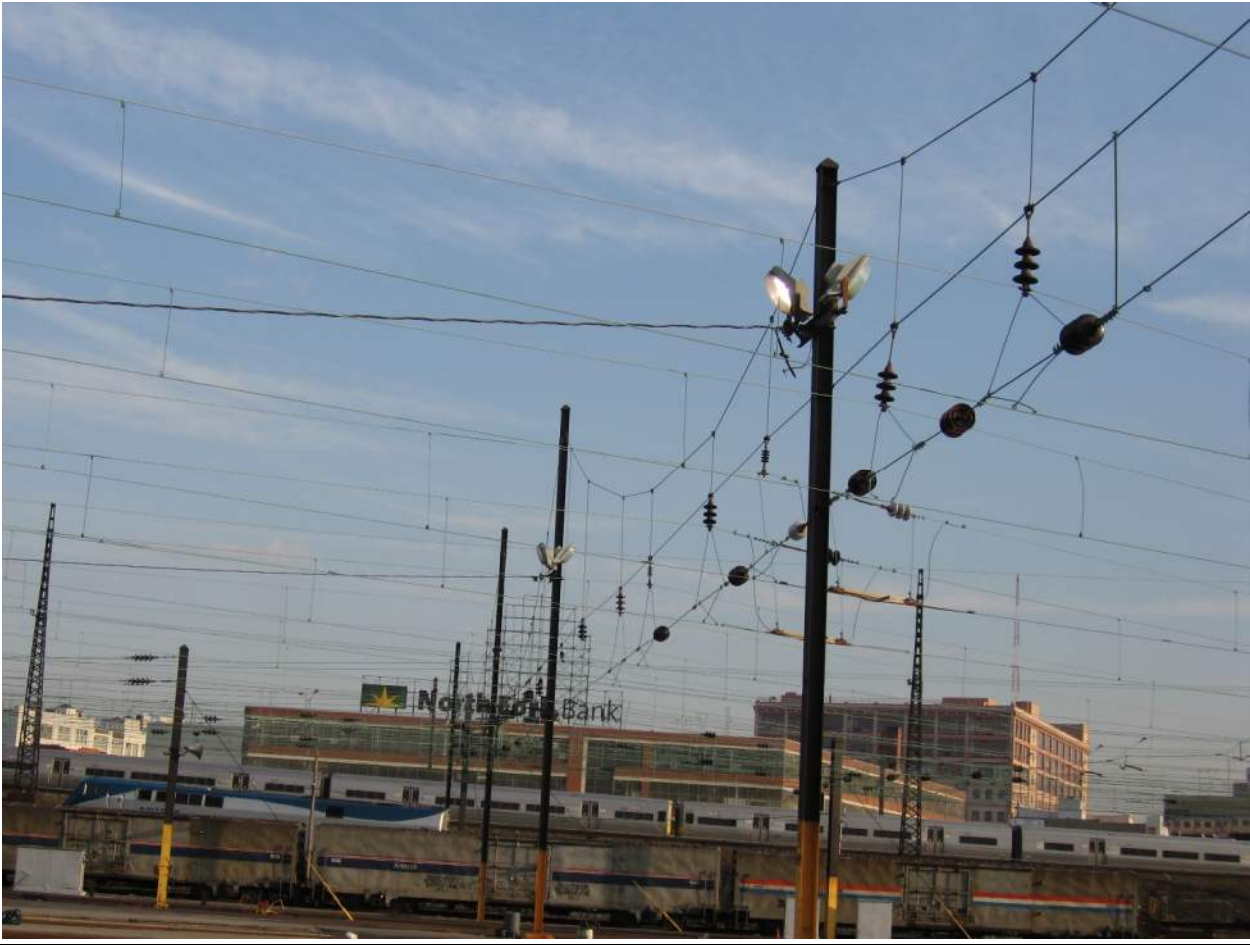
Zone 3 – X Catenary Structure (2):
