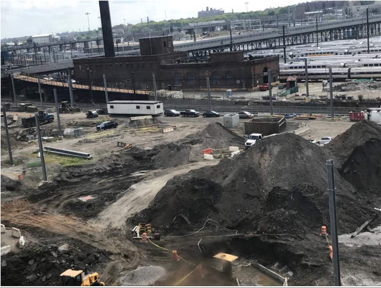
Zone 1 – Lighting Poles (under construction):
