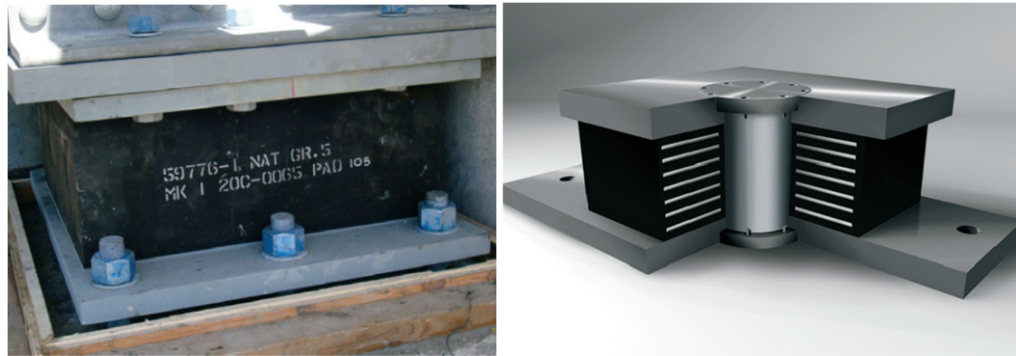
Figure 18 – Lead Core Rubber Bearing
