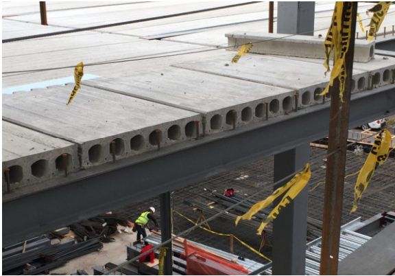
Figure 11 - Standard Rolled WF Beam + Precast Plank
