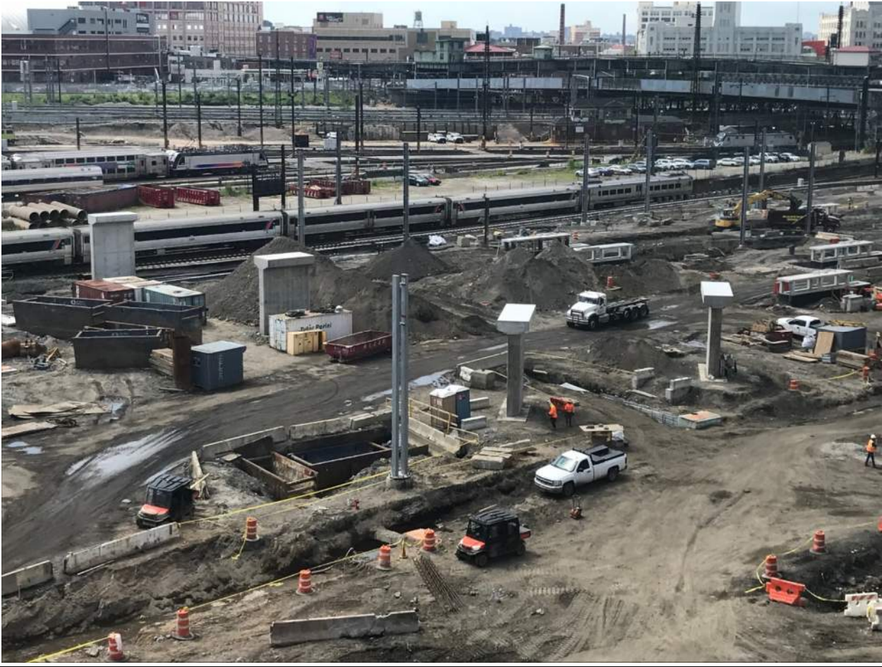
Zone 1 – Pedestrian Bridge (under construction):
