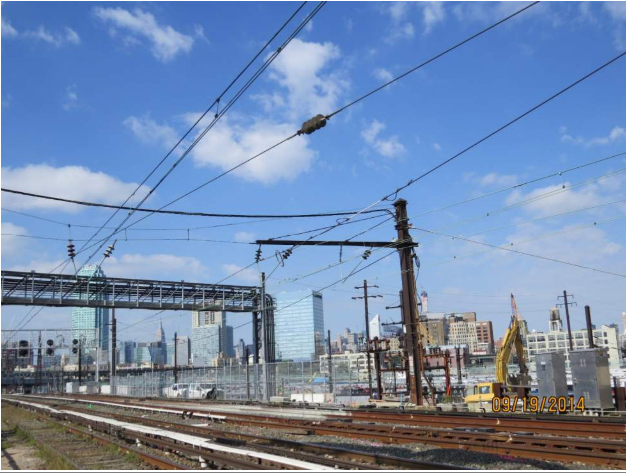
Zone 7 – Aerial Utility Crossing:
