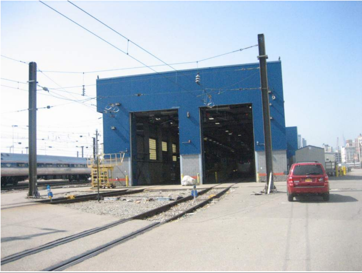
Zone 2 – X Catenary + High Speed Shop:
