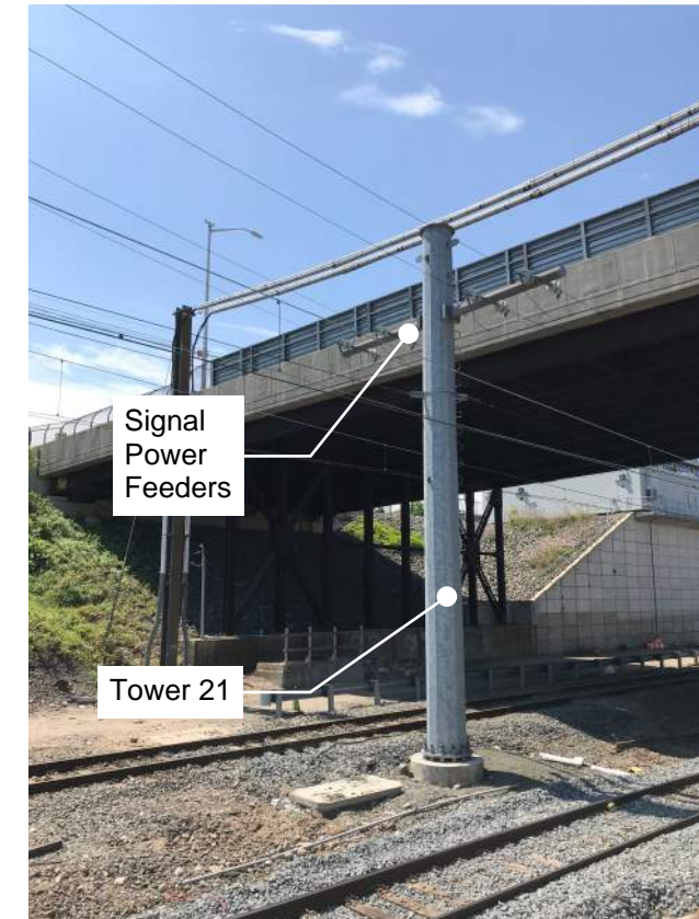
Photo 16 - Feeder circuits
