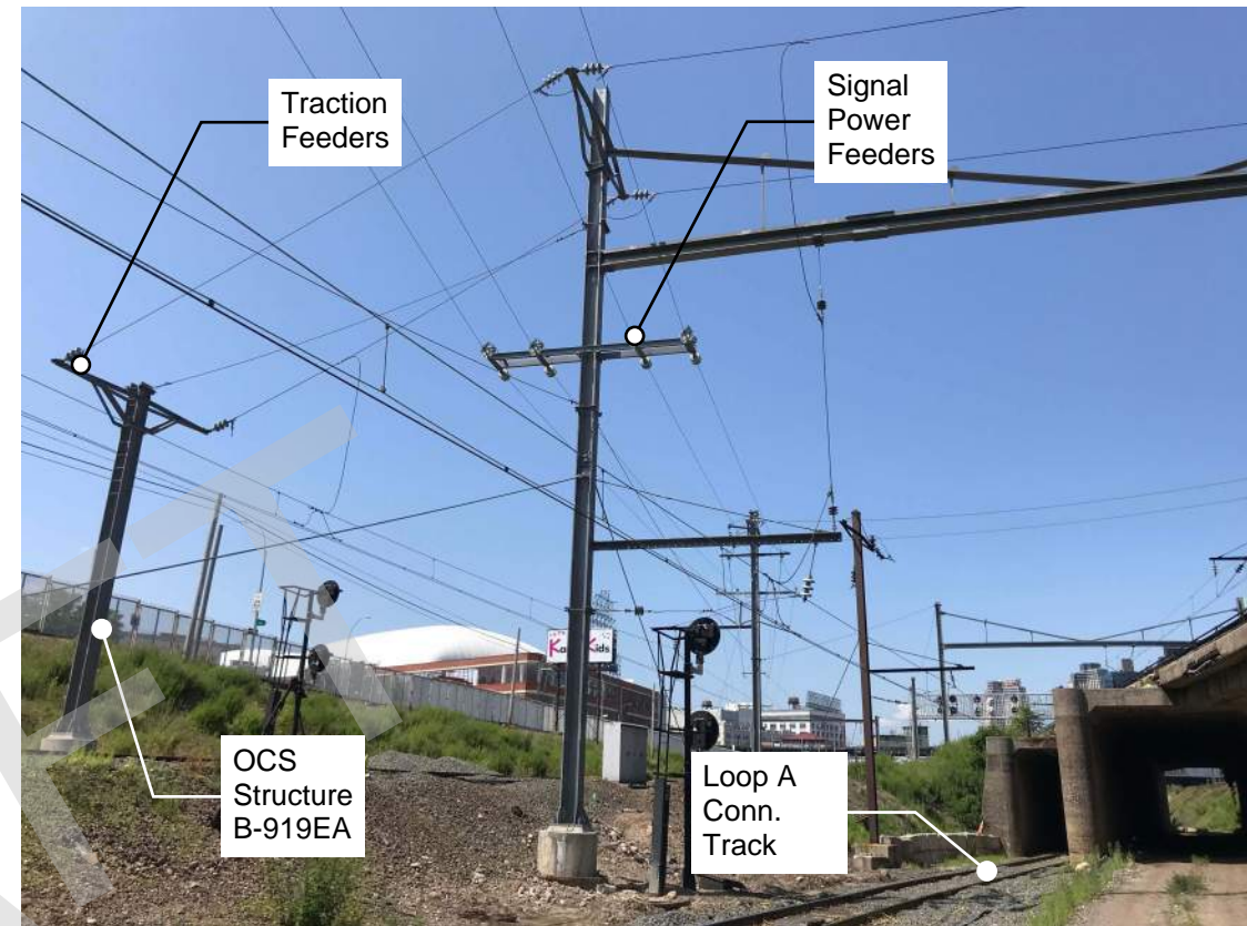
Photo 14 - Feeder Circuits
