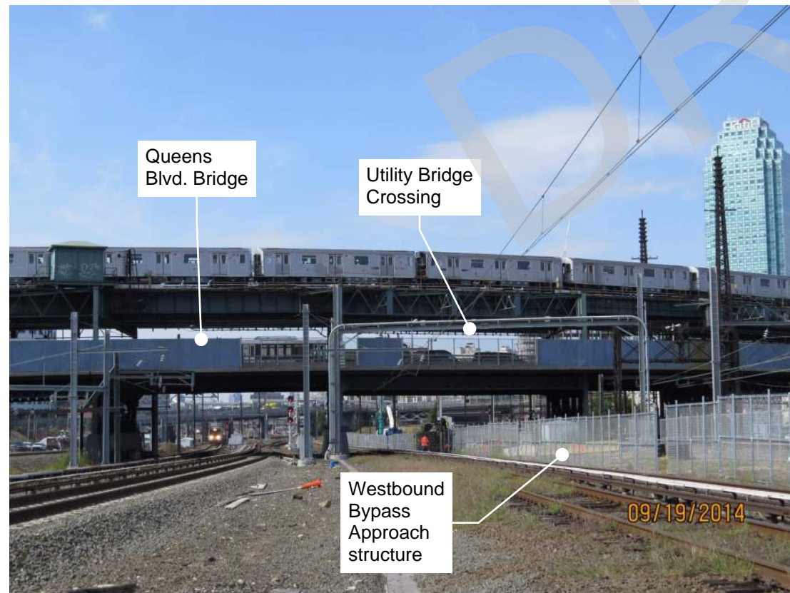
Photo 11 - Aerial Utility Crossing
